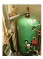
Connect the return DN16 2-in-2 pipe (the one carrying fluid back to the collector) to the top connection of the pump station using a PAW self seal nipple and the back nut – black rubber seal facing towards the pump station.
